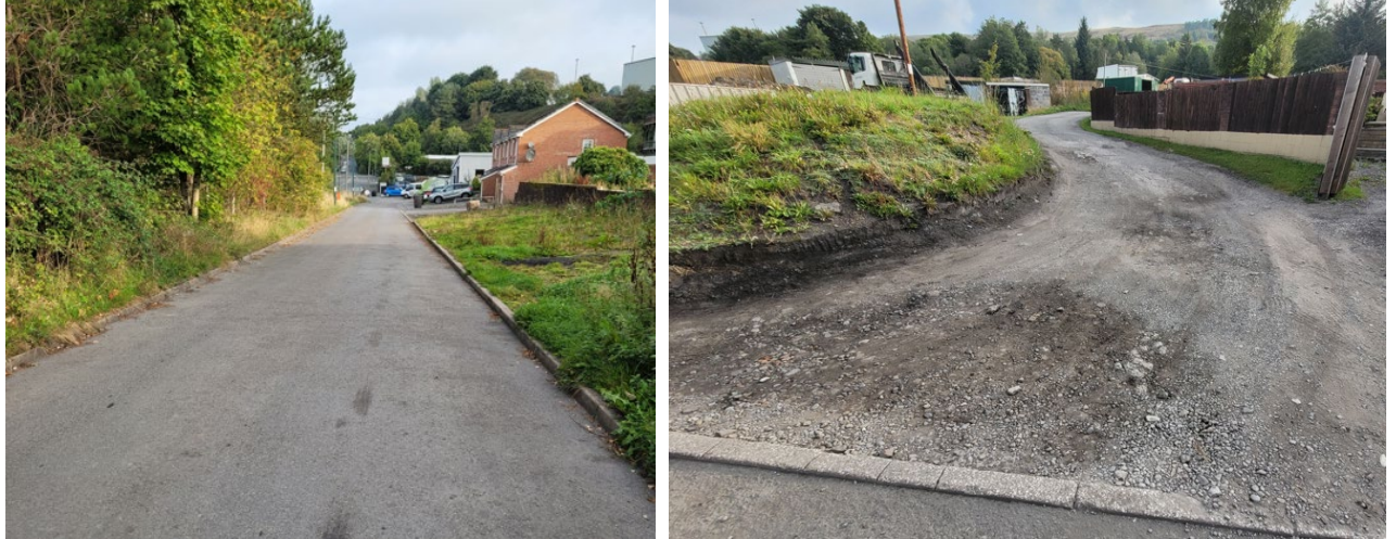
Fig's 11 & 12 (above, L-R) Access road looking northwards and access track leading from the highway in an easterly direction
